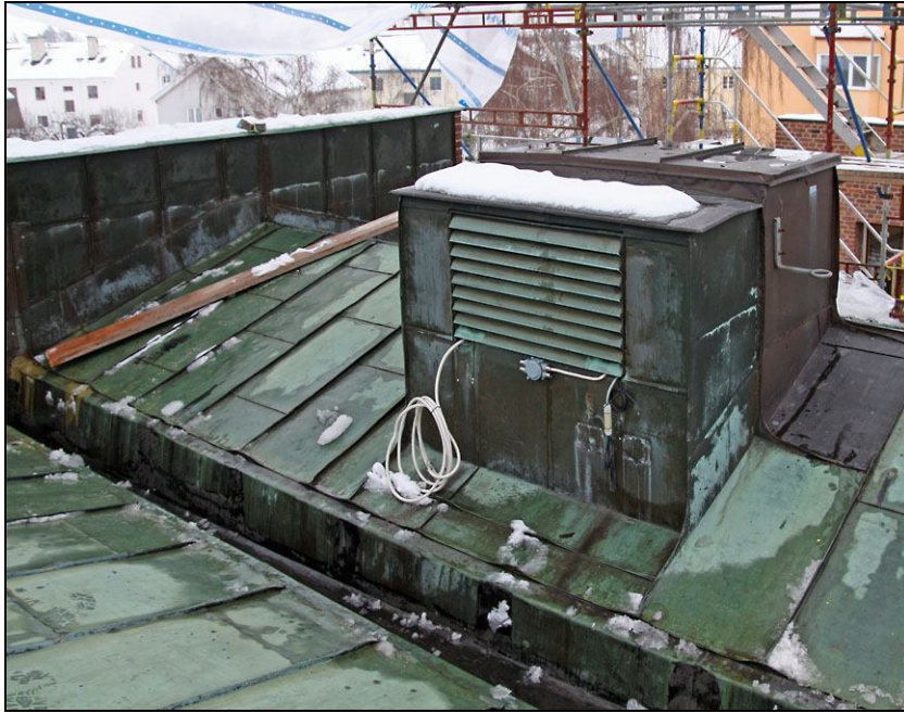
Two fläkthuvor (ventilators) on the north-eastern part of the roof. The hood closest to the image is presumably original, while the one further away has been added in a later stage.
