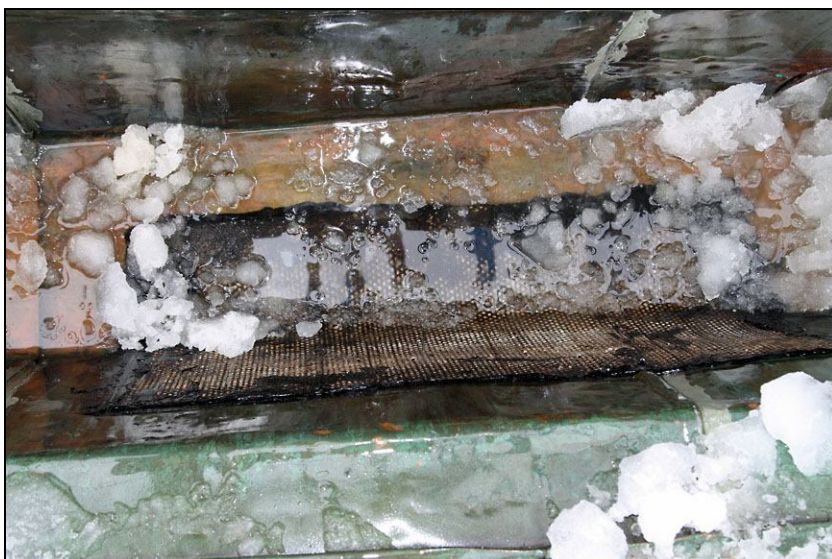
The roof had many temporary coverings. Here, a leak in the gutter was sealed with asphalt putty, which was reinforced with a mesh.
