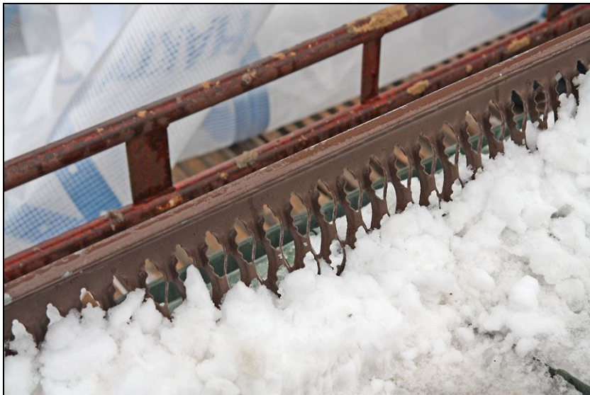
Snow guard at the edge of the roof.
