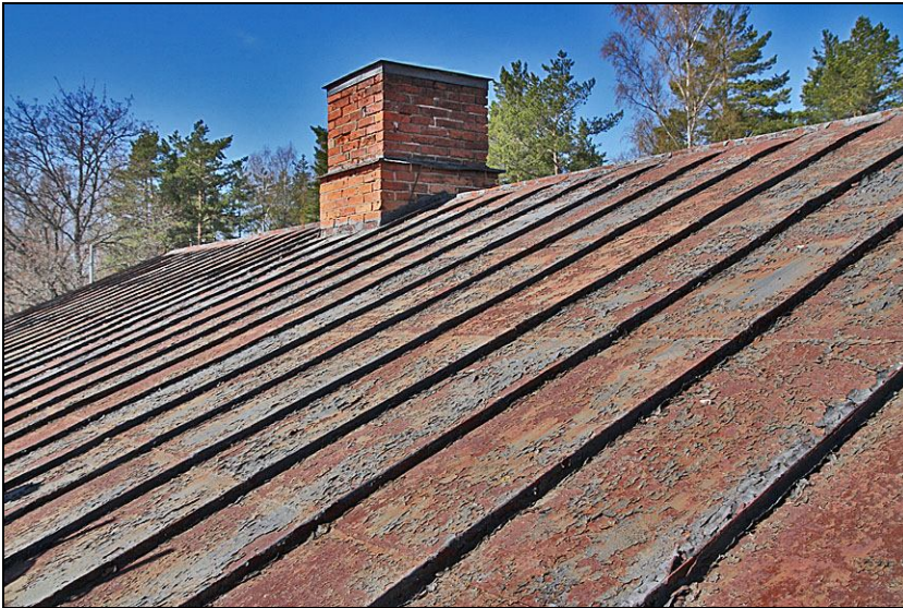
2010-05-07. Skorstenen innan restaurering.
